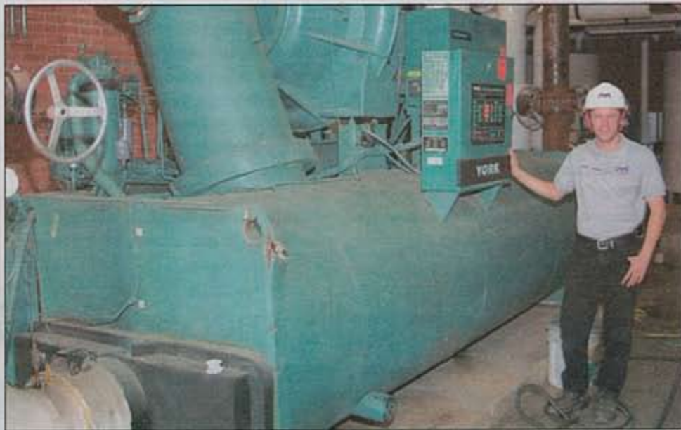
Dave Wallace of Rapid Recovery recovers refrigerant from a chiller.
