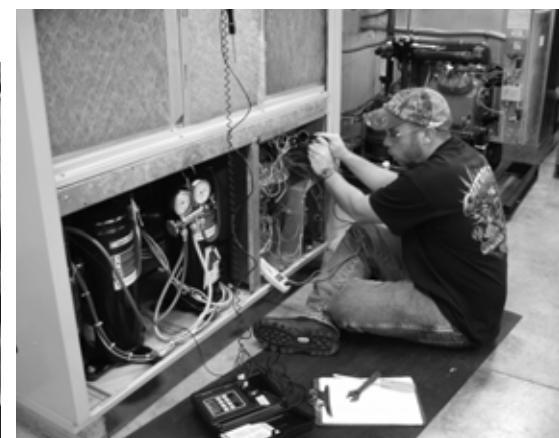
Scotty Osborne checking 10-ton water-cooled air conditioning unit
